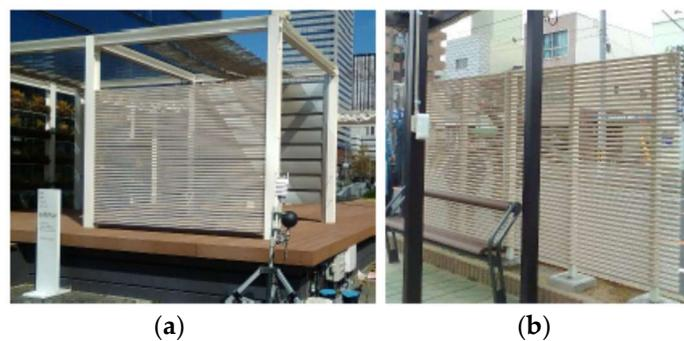
**Figure 3.** Evaporative cooling louver, which is provided by Prof. Misaka. (a) in a park; (b) at a tram stop.
