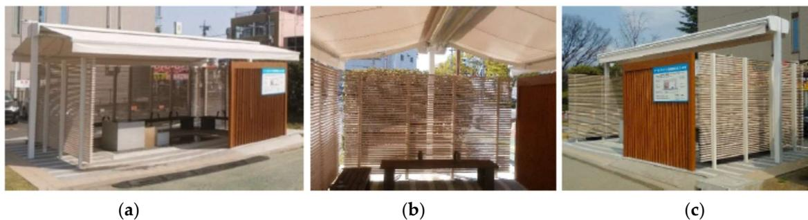
**Figure 1.** Automatically opening and closing awning installed at a bus stop, which are provided by Prof. Misaka. (a) whole view; (b) internal view; (c) closed state.
