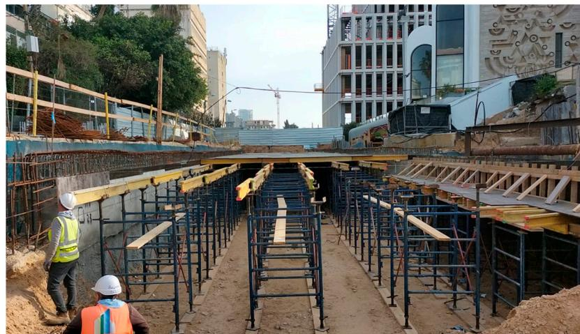
**Figure 2.** Formwork for the tunnel concrete slab during stage 1 of the top-down construction.
