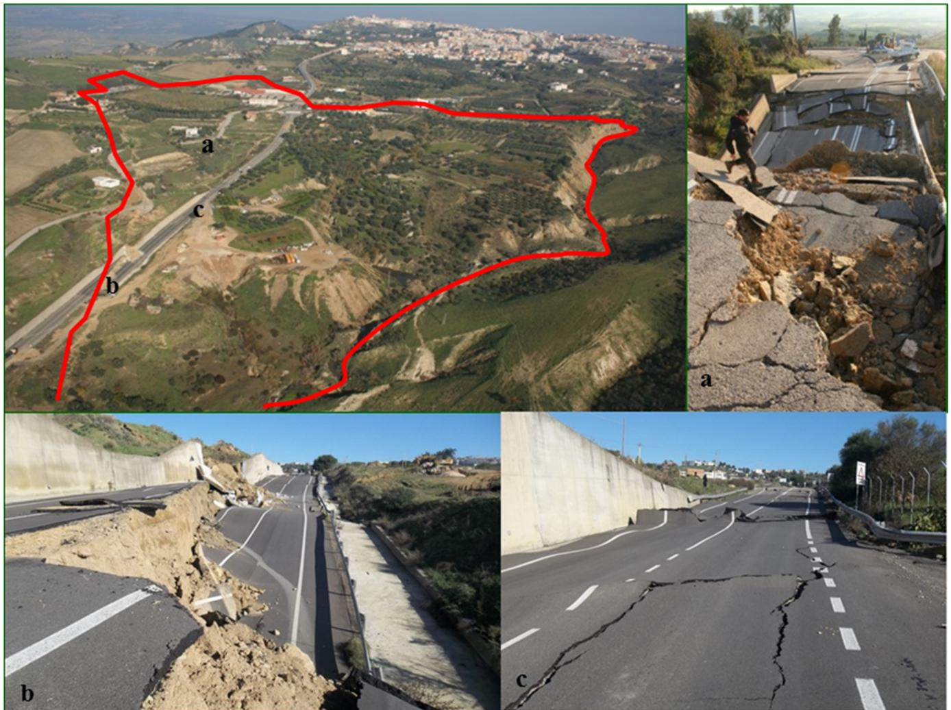
**Figure 2.** Aerial view of the landslide area and some of the most relevant damage to the infrastructures in the affected area. Labels (a, b, c) indicate the location of the pictures in the aerial view.
