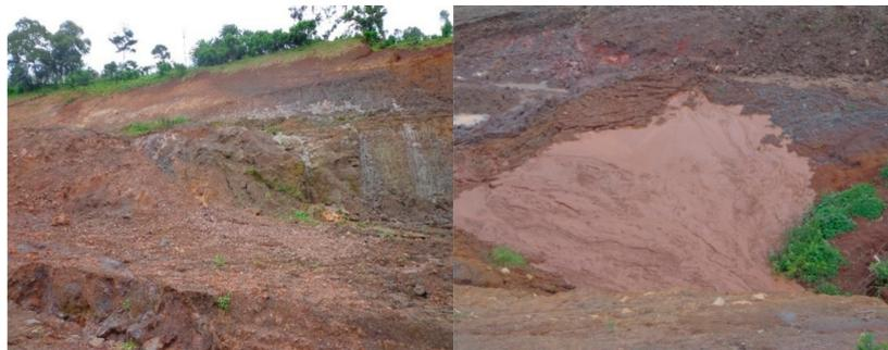
Figure 1. Mode of failure of study area, earth slide (left) and mudflow (right).
