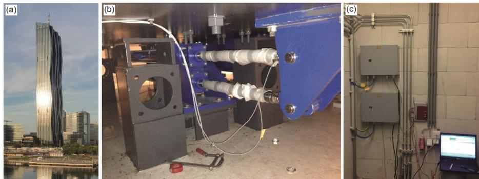
**Figure 18.** (a) Danube City Tower in Vienna, Austria; (b) MR-SVA of Danube City Tower with two controlled MR dampers and (c) two independent real-time controllers.
