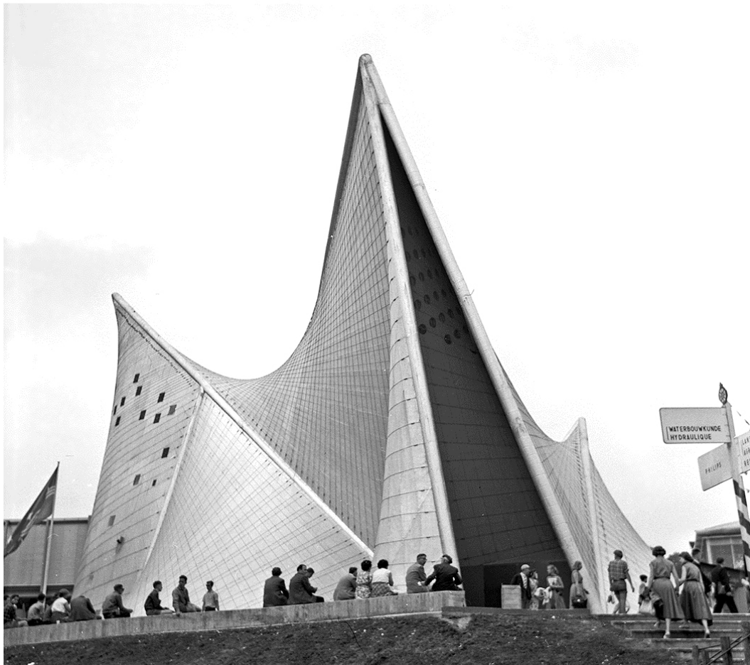
Figure 2. Hyperbolic paraboloids in Iannis Xenakis' sketch for Metastaseis and his design for the Philips Pavilion. Metastaseis sketch from Iannis Xenakis, Formalized Music . Stuyvesant, NY: Pendragon Press, 1996. Philips Pavilion image reprinted under CC BY-SA 3.0 https://creativecommons.org/licenses/by-sa/3.0 via Wikimedia Commons, Wouter Hagens, 1958 (accessed on 5 April 2024).
