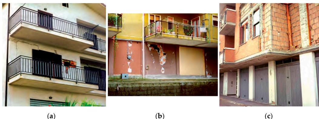
**Figure 2.** Examples of Medium-Severe and Very Heavy damage to infills: horizontal and vertical cracks between infill and beams/columns—widespread damage D2–D3 and locally D4–D5 (a); damage D4–D5 to infills (b); damage D4–D5 with out-of-plane collapse of one infill leaf (c)—adapted from [4].
