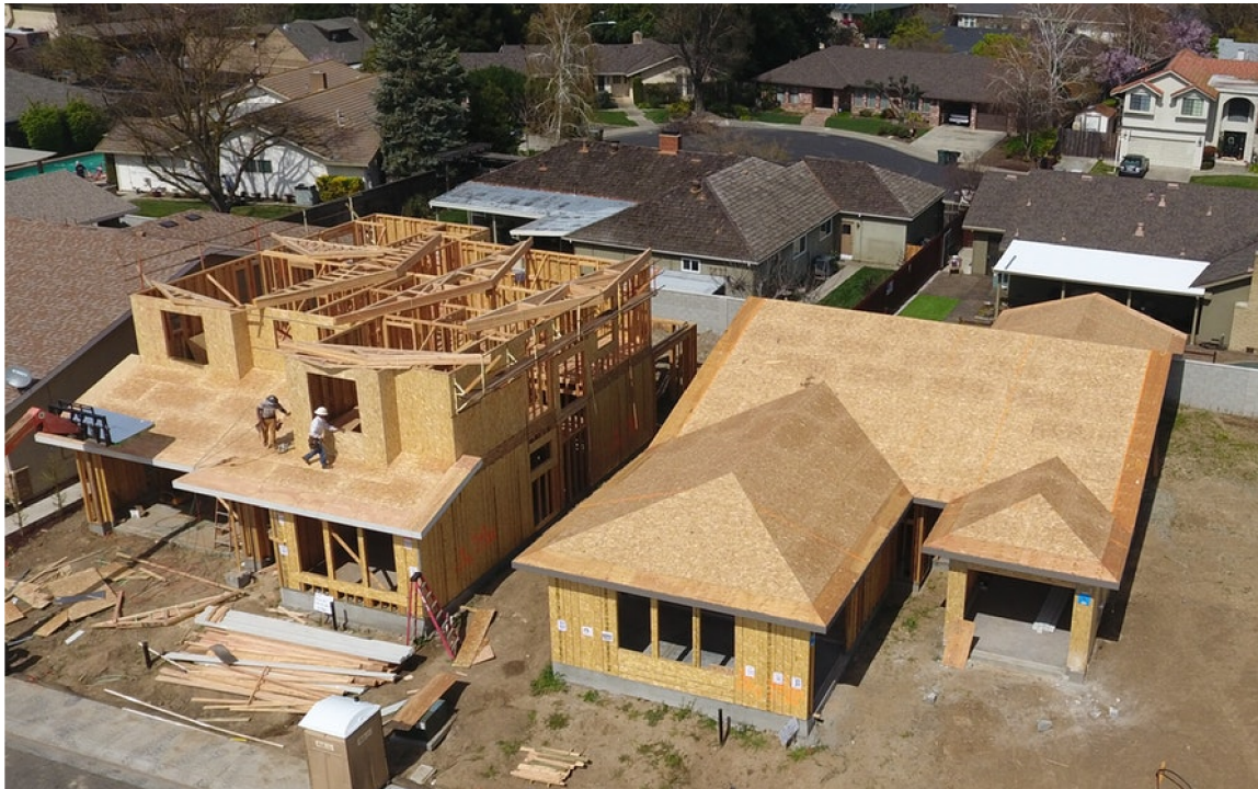
Figure 3. Installation of the OSB-PU SIPs (Source: By Scott Blake https://unsplash.com/photos/3tjM7Un881A ).
