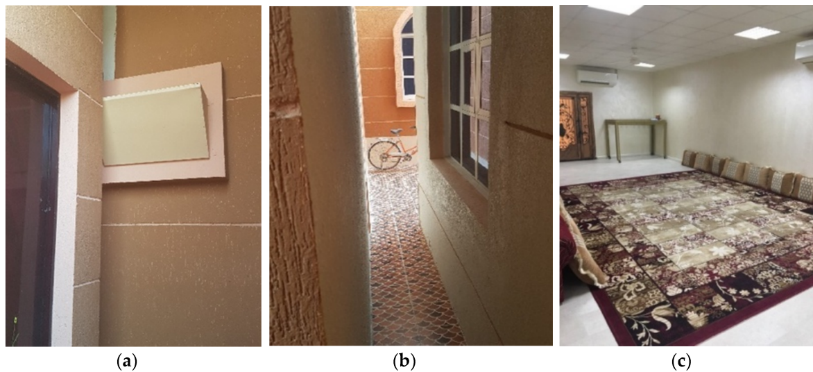
Figure 2. Examples of residents' adaptations of their houses: (a) The extension was too close to the existing part, so the residents were forced to close the bathroom's window for privacy purposes, leaving the bathroom almost without ventilation. (b) The new extended part is located less than 1 m away from the existing house; hence, the window became useless. (c) The residents developed a new living room located in the middle of the ground floor, and it has no windows, so there is no natural lighting or ventilation.
