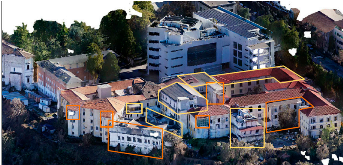
Figure 8. Identification of inadequate additions (yellow outlines) or design incongruity (orange outlines) that have to be demolished: the technologies used for the investigations allowed to carry out highly detailed studies on volumes, in order to accurately determine the configuration of the building for the project initial phase.
