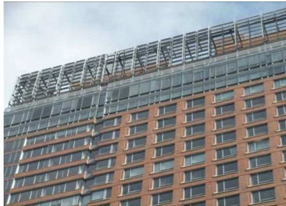
**Figure 8.** The Riverhouse dynamic PV system [28].
