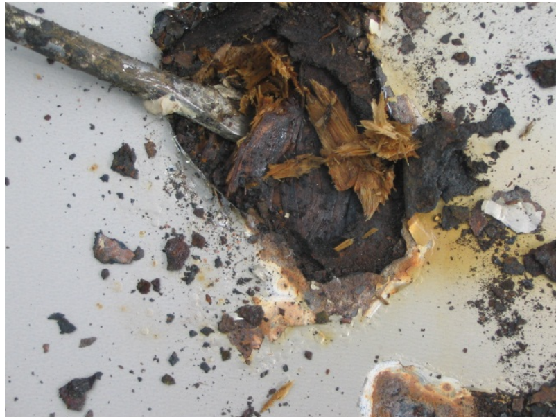
Figure 4. Deterioration of oriented strand board (OSB) at roof.
