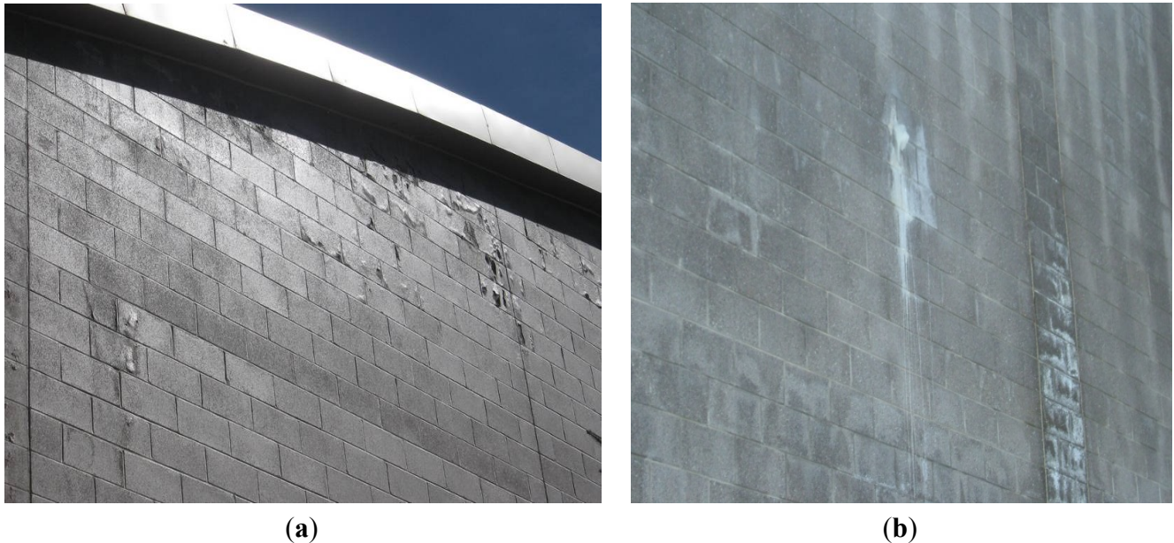
Figure 2. (a) Blistering and spalling at south façade; (b) Ice formations.
