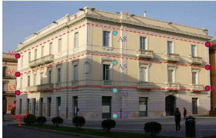
Different sets of accelerometric recordings are available caused by ambient noise and impulsive sources (*i.e.*, the fall of 1 m<sup>3</sup> concrete block on a truck placed close to the building, the rapid braking of the truck along the Y direction of the building, some knocks of an instrumented hammer).
