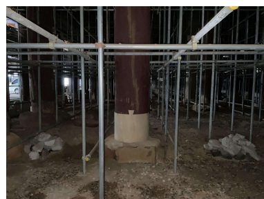
Figure 7. Repairing the lower part of a column. According to the principle of preserving the original, the whole column is not replaced, but only the damaged part is cut out, and a new one of the same shape is made. This is a common method for repairing a hanok. (National treasure: Yeosu Jinnamgwan.).
