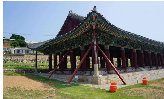
Figure 1. Steel supports to prevent the column leaning phenomenon. This hanok's columns were leaning outward, and steel supports were installed to prevent further leaning. As of 2016, the hanok has been completely dismantled and repaired. The cause is unknown. (National treasure: Yeosu Jinnamgwan).
