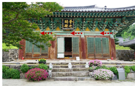
Figure 2. Columns leaning to the left. The upper part of the column is visibly leaning to the left. The cause remains unknown. (Treasure: Wanju Wibongsa Bogwangmyeongjeon, taken in 2018).
