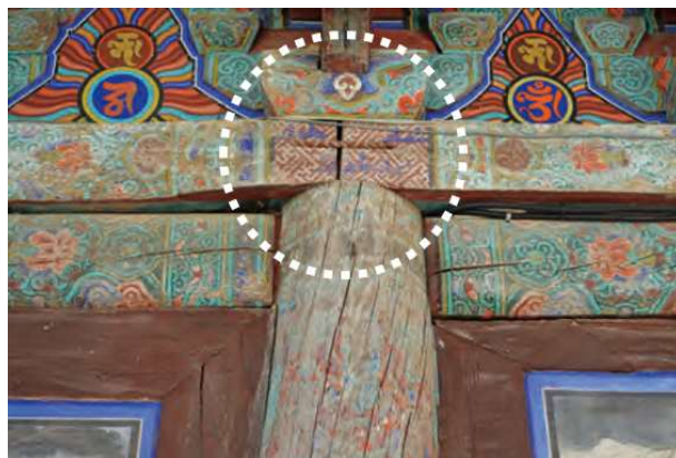
Figure 59. Pyeongbang. Pyeongbang is a horizontal member placed on an external column. This is an example of reinforcing the joints with “C”-shaped steel (white circle) to prevent the pyeongbangs from separating. (Treasure: Daegu pagyesa wontongjeon).
