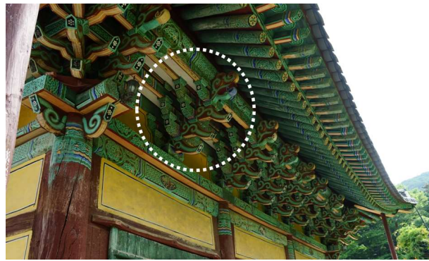
Figure 20. The style of Gongpo: Dapo. The Dapo style (white circle) is the most splendid. In the same form as Jusimpo, a Gongpo is added to the top of a horizontal member between columns. It is mainly found in palace and temple buildings.
