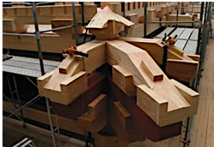
Figure 23. The replacement timbers are assembled in their final positions using traditional techniques (Nara 2006).
