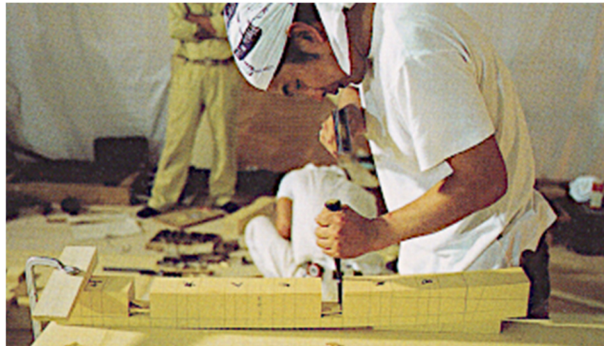
Figure 18. Re-prototyping of the timbers according to old carpenters' manuals.
