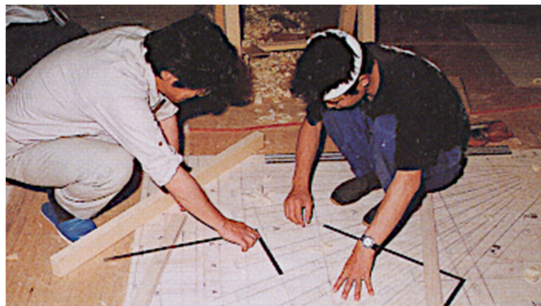
Figure 17. Decoding traditional design methods, based on old carpenters’ manuals.
