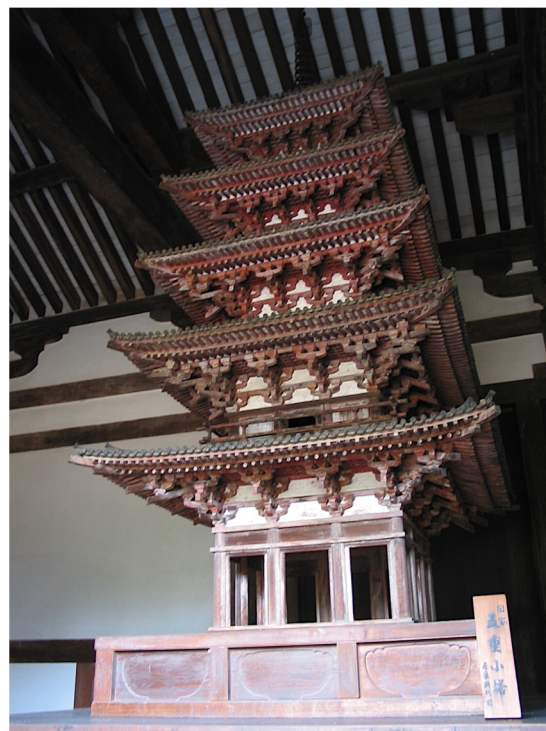
Figure 25. The remaining original 1/5 scale design model (a small five-floor tower) of Kairyuouji Pagoda, Japan.
