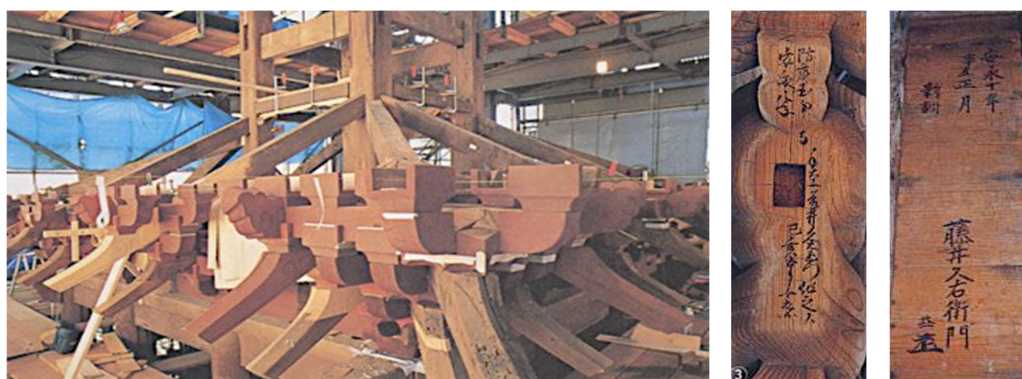
Figure 38. Replacement of decayed timbers with new ones in their original positions and with their original function, conserving the original components by using traditional jointing techniques and saving the historical information written in ink on the wood (Nara, 2004).
