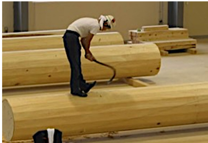
Figure 22. Using authentic materials (Hinoki wood) and traditional carpentry tools to recreate the historical aspect of replacement timbers (Nara 2006).
