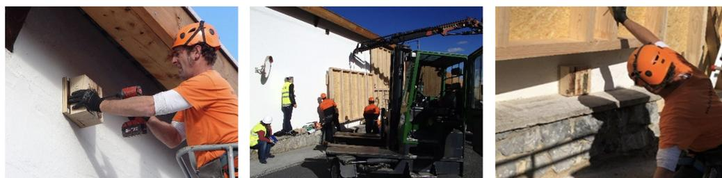
Figure 19. Installation sequence of the modules. The module below installed with a crane.
