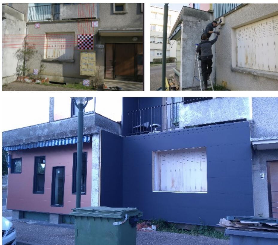
**Figure 22.** First achievements with photogrammetry and a module installed with an MK concept in a real project. Bottom picture by Mr Hervé Coperet (POBI Industrie).
