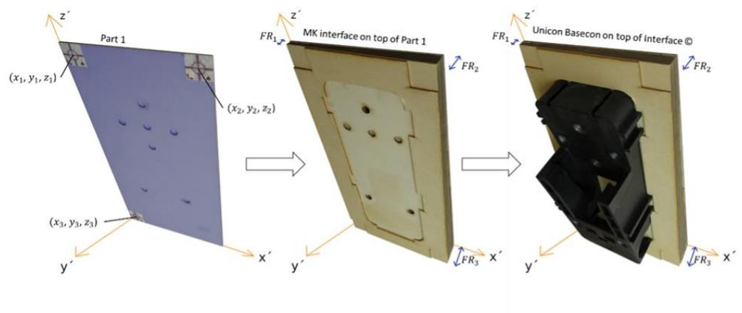
Figure 9. Three phases for installing the MK on top of the building facade.
