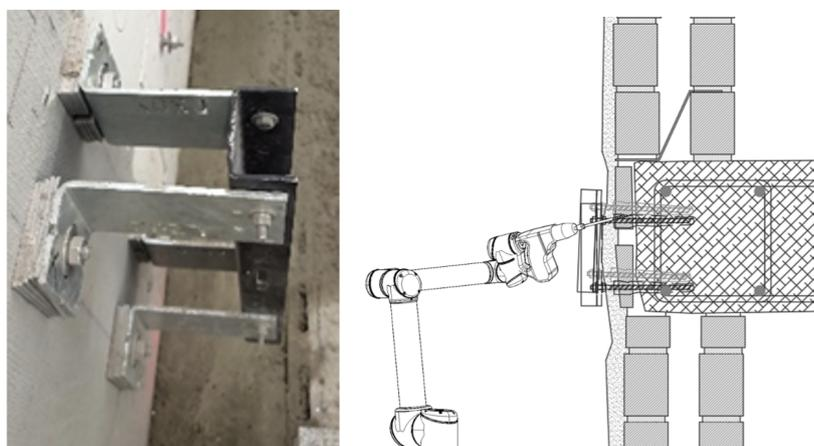
**Figure 4.** Left: accurately placed connector for rain-screen by using several wedges. Right: deviations occur while drilling and placing, manually or with robots.
