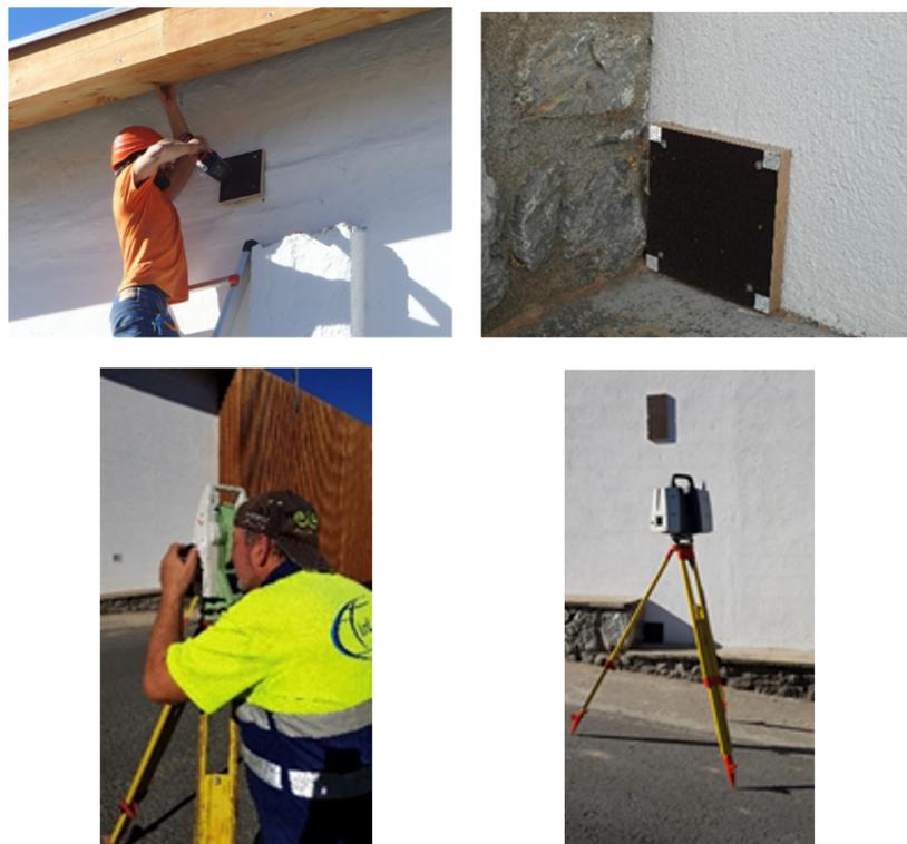
**Figure 16.** Top left and right: fixation of Part 1. Bottom left: point survey using Total Station. Bottom right: laser scanner at work.
