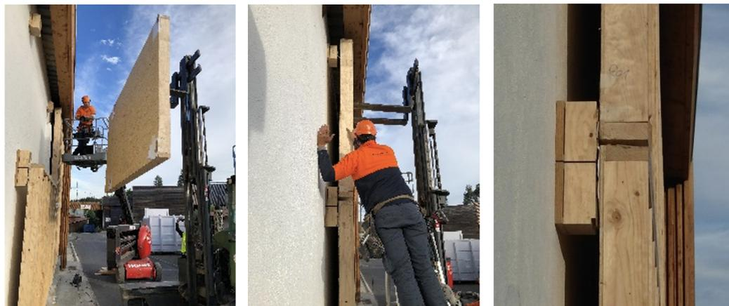
Figure 20. Installation sequence of the modules.
