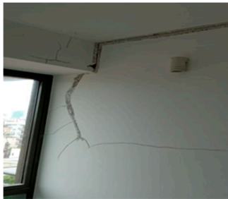
(j) Wall crack
