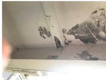
(h) Concrete spalling
