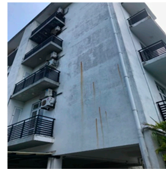
(f) Wall staining due to corroded steel
