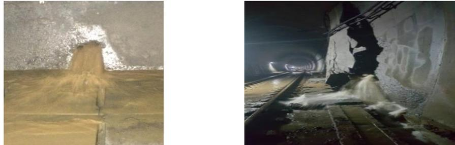
**Figure 1.** A typical site of water damage in a tunnel.
