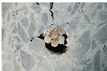
**Figure 24.** Example of discontinuity of cover around prestressing strings and void located in concrete cover.
