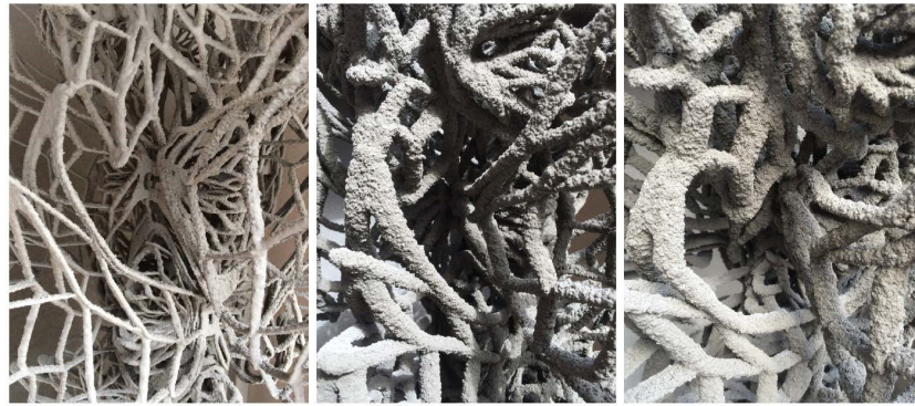
Figure 19. The process of spraying the cement (layer by layer) onto the steel skeleton, and the granular texture is shown on the surface of the cement mixture.
