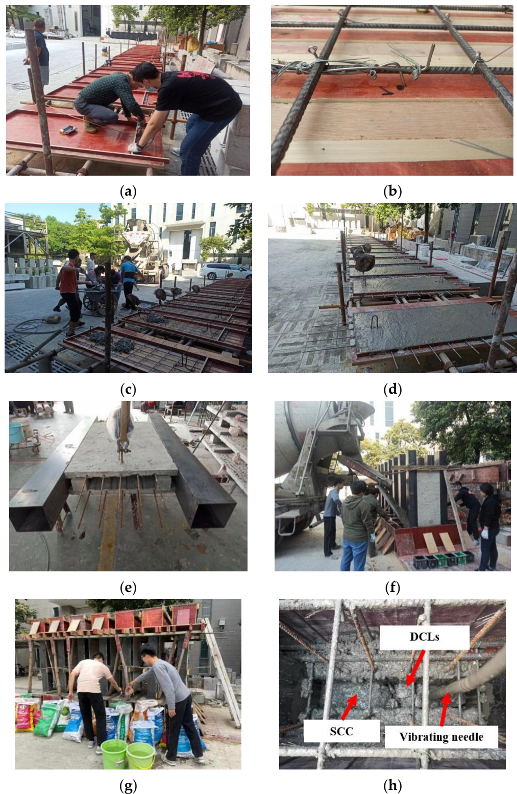
Figure 2. Concrete casting of specimens. (a) Formwork; (b) Thermocouple arrangement; (c) Precast wallboard pouring; (d) Precast wallboard pouring completed; (e) Precast wallboard and steel pipe assembling; (f) Casting of foundation beam; (g) Wet DCLs; (h) Cavity pouring. The variables studied experimentally included fire exposure time, fire-retardant coating on the edge constraint steel pipe column, and the width-thickness ratio. The basic parameters of each specimen are detailed in Table 1.
