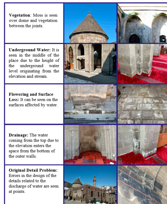
Figure 10. Damages observed in the Ulu Mosque.
