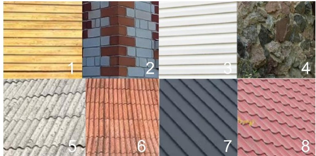
Figure 14. Building materials of garden houses: 1—wooden cladding, 2—bricks, 3—plastic boards, 4—field stones, 5—gray asbestos panels, 6—pink asbestos panels, 7—rolled tin, 8—steel sheets. Photos by A. Gabrėnas.
