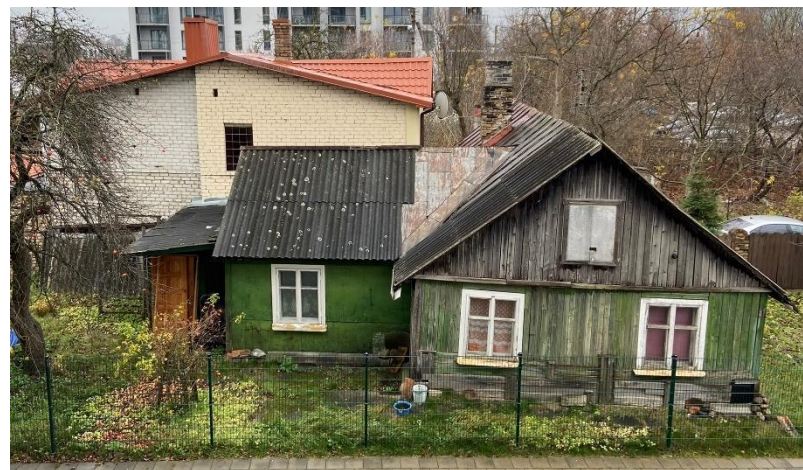
Figure 8. Building in green color: wall—metal sheet, wooden cladding, roof—asbestos, rolled tin. Building in white color: wall—bricks, roof—steel. Photo by A. Gabrėnas.
