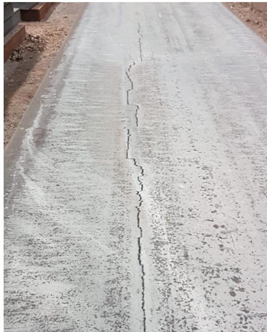
**Figure 1.** Example of a visible longitudinal crack.
