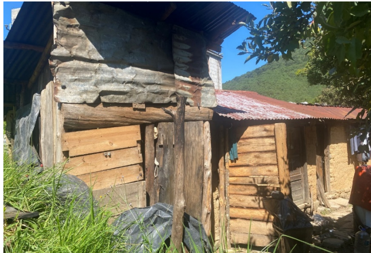
Figure 8. Utilization of reused metal sheets with perforations and deformations.
