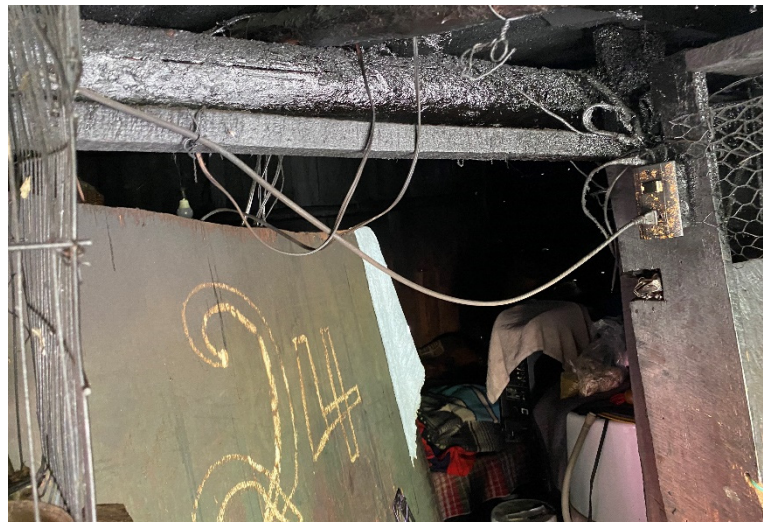
Figure 6. Wooden elements inside the house show grease adherence.
