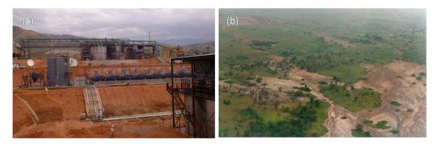
**Figure 7.** Bioleaching plant (**a**) for the processing of pyritic tailings (**b**) containing cobalt, copper, nickel and zinc. Photographs from D. Morin, Bureau de Recherches Géologiques et Minières (BRGM), reprinted with permission.
