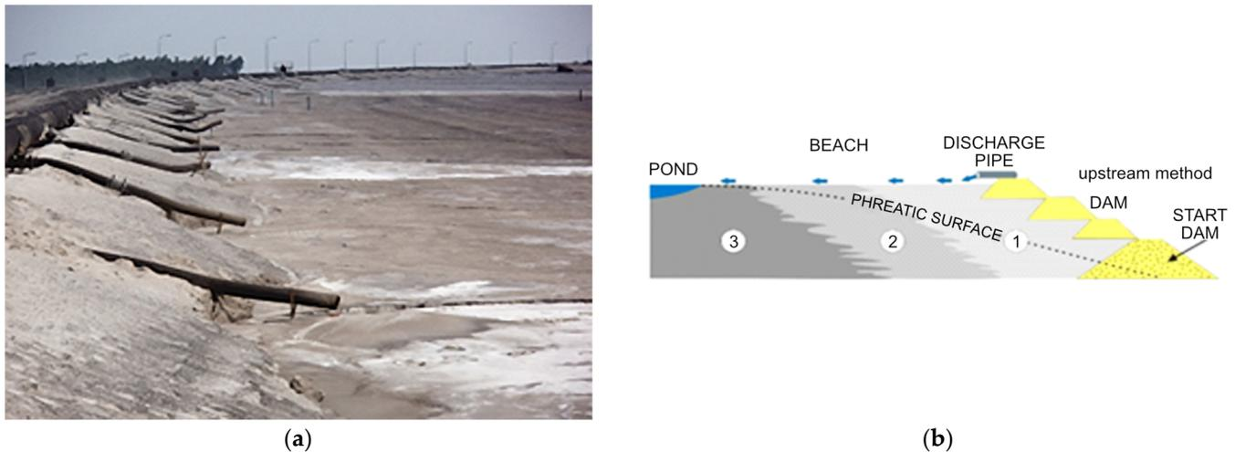
**Figure 2.** Żelazny Most TSF: (a) wet deposition of tailings, photo: KGHM Polska Miedź; (b) diagrammatic section: 1—coarse tailings (fine sands), 2—transitional zone (silt and sand), 3—fine tailings and slimes (clay and silt) [1].
