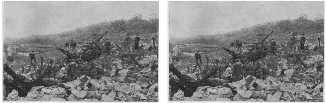
**Figure 13.** The landslide body (left, right) and the damage caused to a retaining wall (right) (Source: [67], private archive of Gizzi F.T.).
