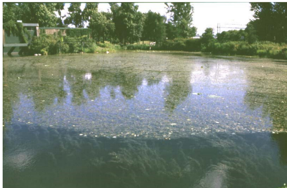
Figure 4. Surface flow CW with submerged macrophytes (mostly Myriophyllum spicatum , water milfoil) in Montréal, Canada. Photo Jan Vymazal.
