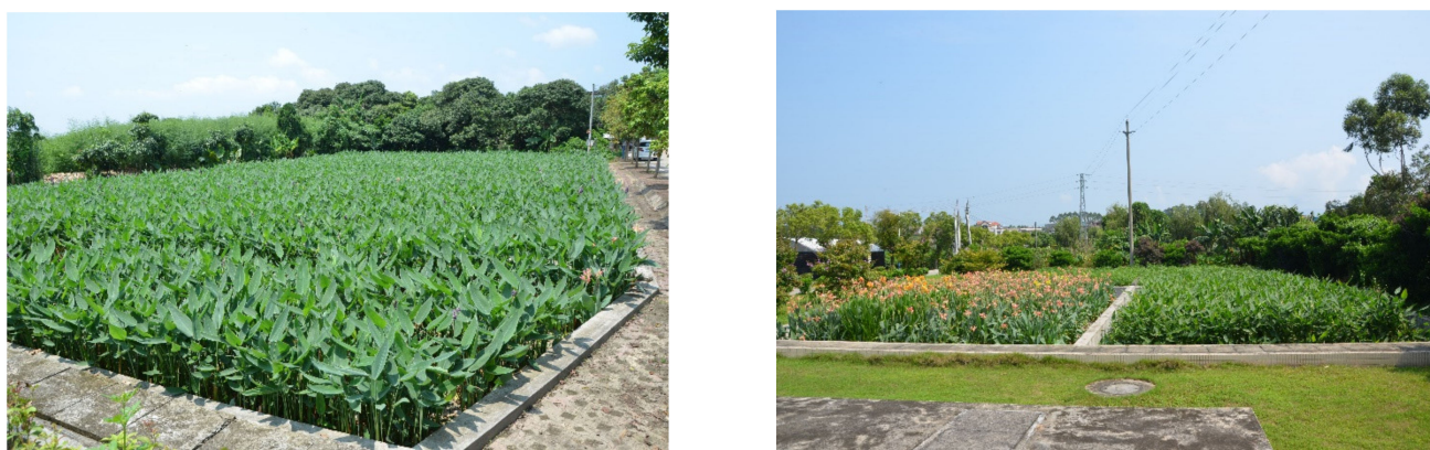
Figure 18. Constructed wetlands with horizontal subsurface flow, planted with Thalia dealbata (left) and Canna indica and Thalia dealbata (right) in Quangdong Province near Guangzhou. Photo Jan Vymazal.
