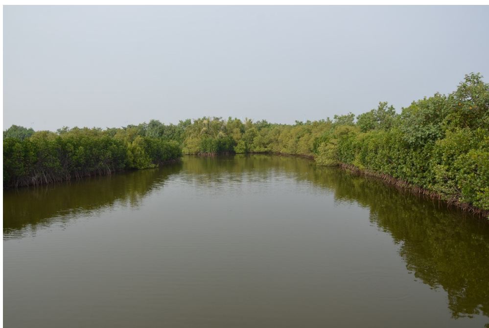
Figure 7. Dapeng Bay, Taiwan: surface flow constructed wetland with mangroves ( Kandelia candel ) for the treatment of mariculture wastewater. Photo Jan Vymazal.
