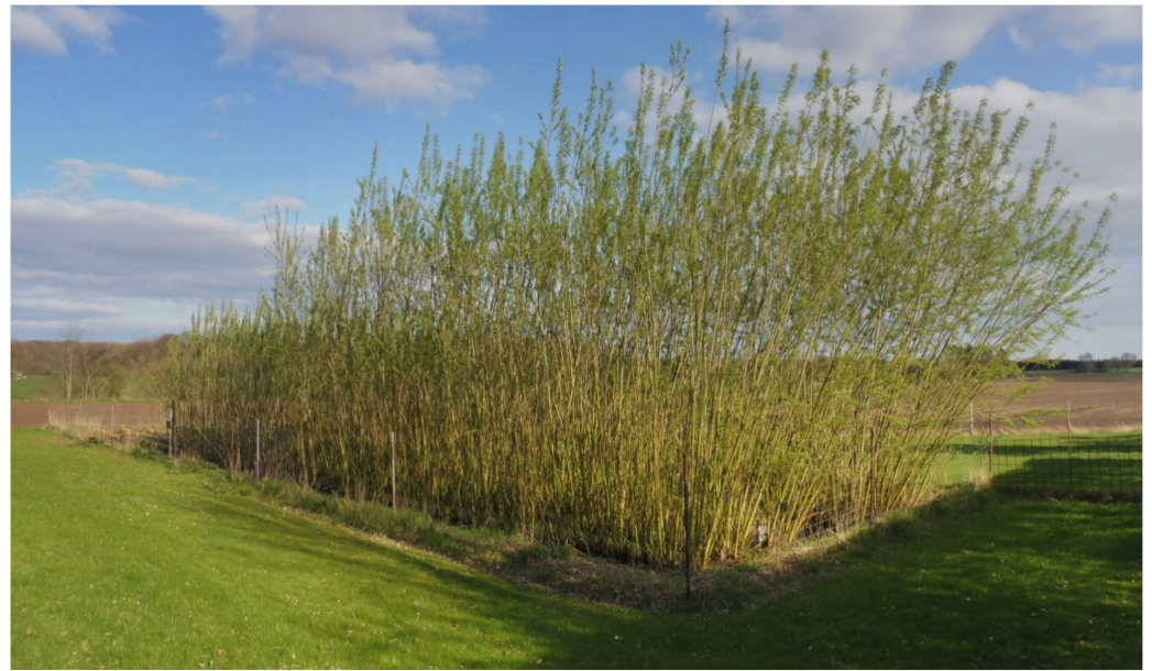
Figure 14. Zero discharge constructed wetlands planted with Salix viminalis (basket willow). Borup, Denmark. Photo Jan Vymazal.
