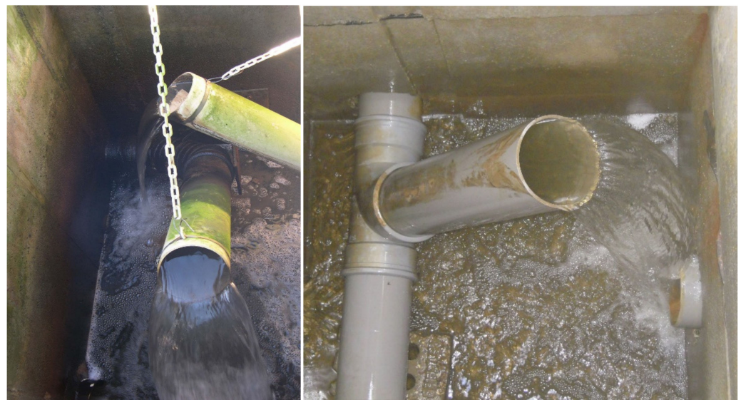
Figure 10. Water level maintenance. Left: outflow pipes hanging on a chain at CW Waikeria, New Zealand. Right: swiveling elbow at CW Bouvron, France. Photo Jan Vymazal.
