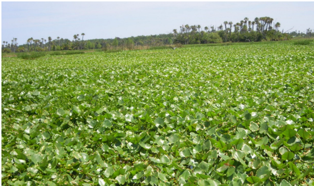
Figure 3. Constructed wetland (Ironbridge, Florida) planted with Nuphar lutea (spatterdock), designed for tertiary treatment of 800,000 PE in Orlando, Florida. Photo Jan Vymazal.
