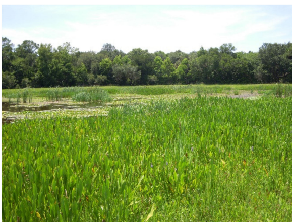
Figure 16. Surface flow CW at Ironbridge. Tertiary treatment for the city of Orlando, Florida. Photo Jan Vymazal.
