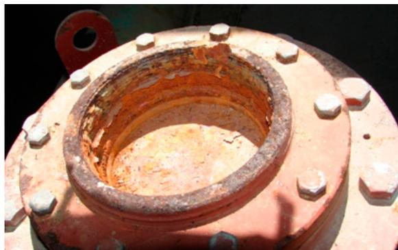
Figure 5. Damage air valve at station 0 + 990.42.
