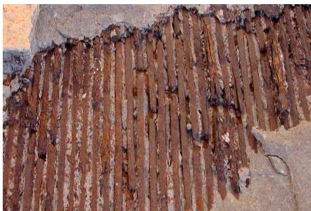
**Figure 4.** Distressed area of a PCCP.
