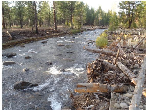
**Figure 9.** Constructed riffle on Whychus Creek, Oregon.
