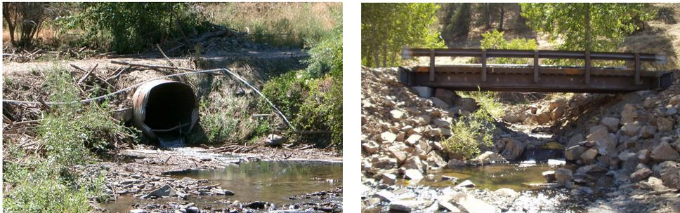
**Figure 1.** Original undersized culvert and subsequent bridge replacement.
