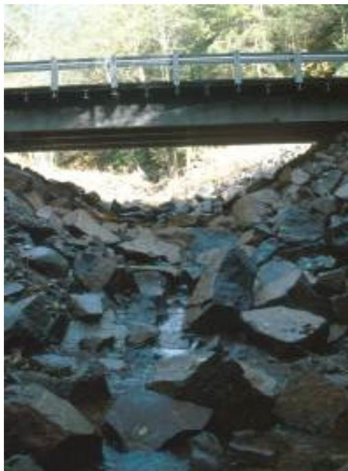
**Figure 13.** Constructed Cascade (photo courtesy of Dan Perritt).
