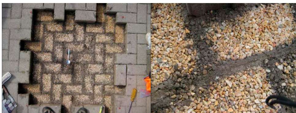
Figure 2. Sediment Accumulation Pattern on Bedding Aggregate [9].
