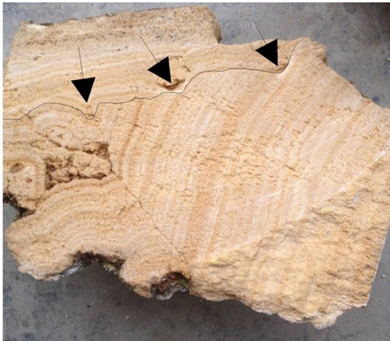
**Figure 12.** Cleaning traces in the aqueduct of Divona, with marks made by a scraping tool (Photo Cees Passchier).
