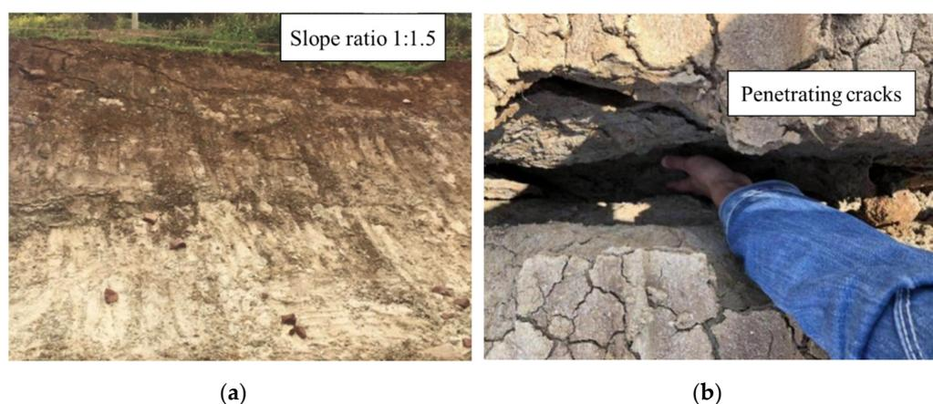
**Figure 2.** Slope failure problem: (a) natural slope with a slope ratio of 1:1.5; (b) penetrating cracks that appear under the alternating action of dry and wet conditions.
