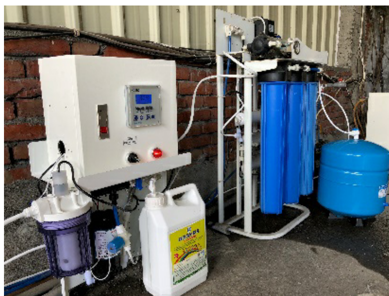
Figure 5. Fully installed water purification and disinfectant system.
