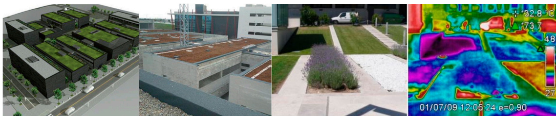
Figure 4. Sustainable drainage urban systems (SUDS) to reduce the urban heat island (UHI). Model and development of green roof on the Parc Bit building, Palma de Mallorca, Spain. Example of thermography to track the UHI evolution.
