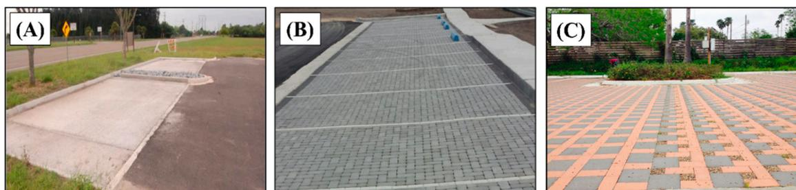
**Figure 1.** Three types of monitored permeable pavements in different parking lots at Lower Rio Grande Valley (LRGV) sites. From the left: (A) Porous Concrete Pavement (PCP), (B) Permeable Interlocking Concrete Pavement (PICP), and (C) Interlocking Block Pavement with Gravel (IBPG).
