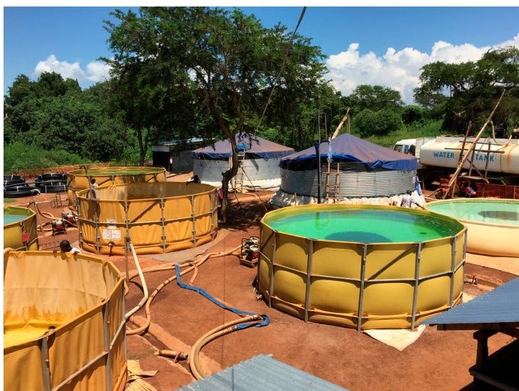
**Figure 1.** Image of multiple clarification tanks, clear tanks, and pumping to tanker trucks at the Palorinya surface-water treatment plant (SWTP), August 2017 (Source: Syed Imran Ali).
