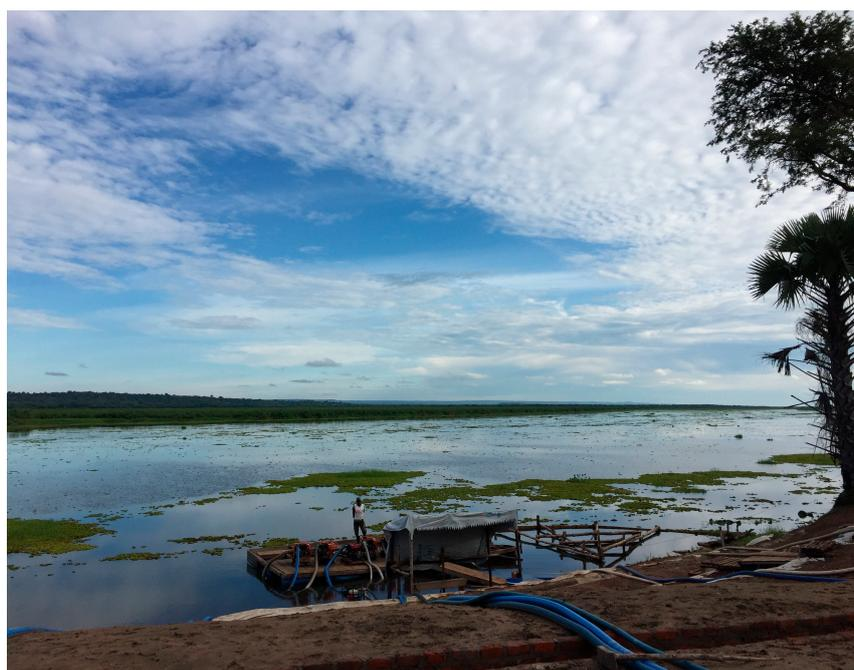
**Figure 3.** Raw water intake from the White Nile at the Palorinya SWTP in August 2017; note marshy condition of river (Source: Syed Imran Ali).
