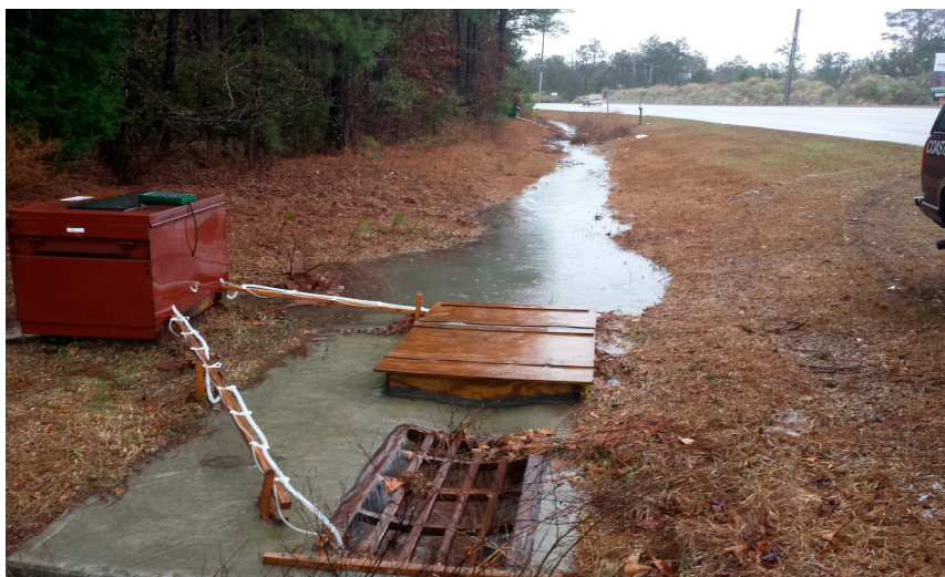
Figure 4. Bioswale outlet structure, with the upstream grate housing the underdrain monitoring and the downstream grate housing the overflow monitoring. The completed bioswale is present in the background.
