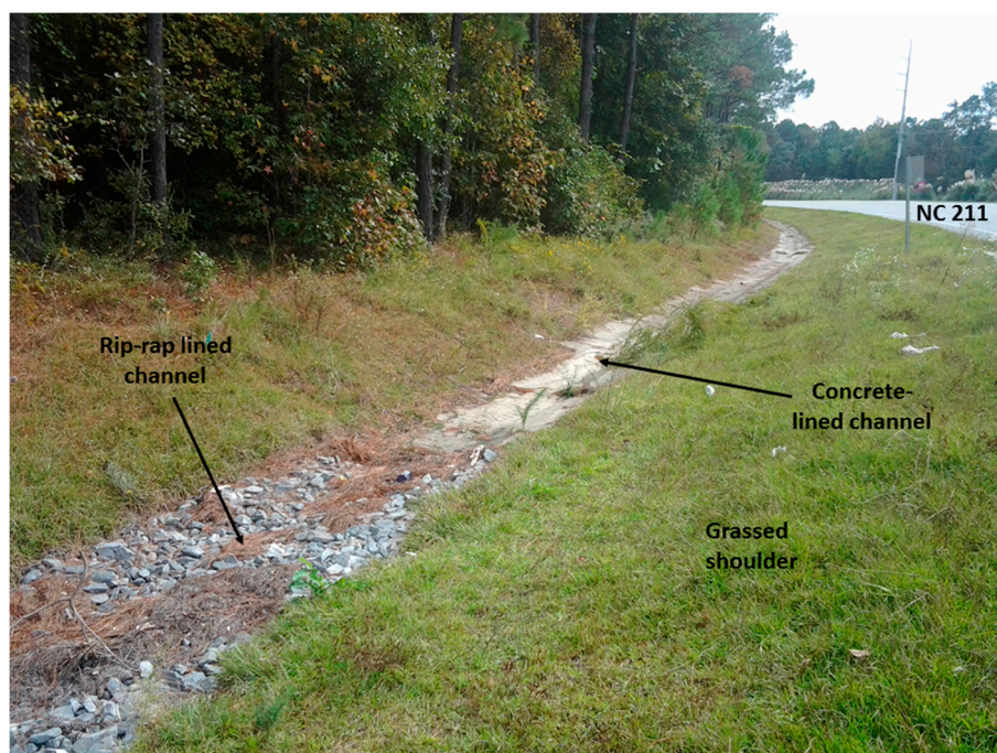
Figure 1. Watershed, grassed shoulder, and concrete-lined channel leading to the forebay of the bioswale.
