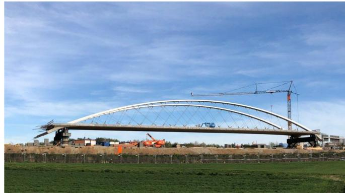
**Figure 1.** Network arch bridge with inclined CFRP cables, reprinted from ref. [9], reproduced with permission by Prof. Urs Meier.
