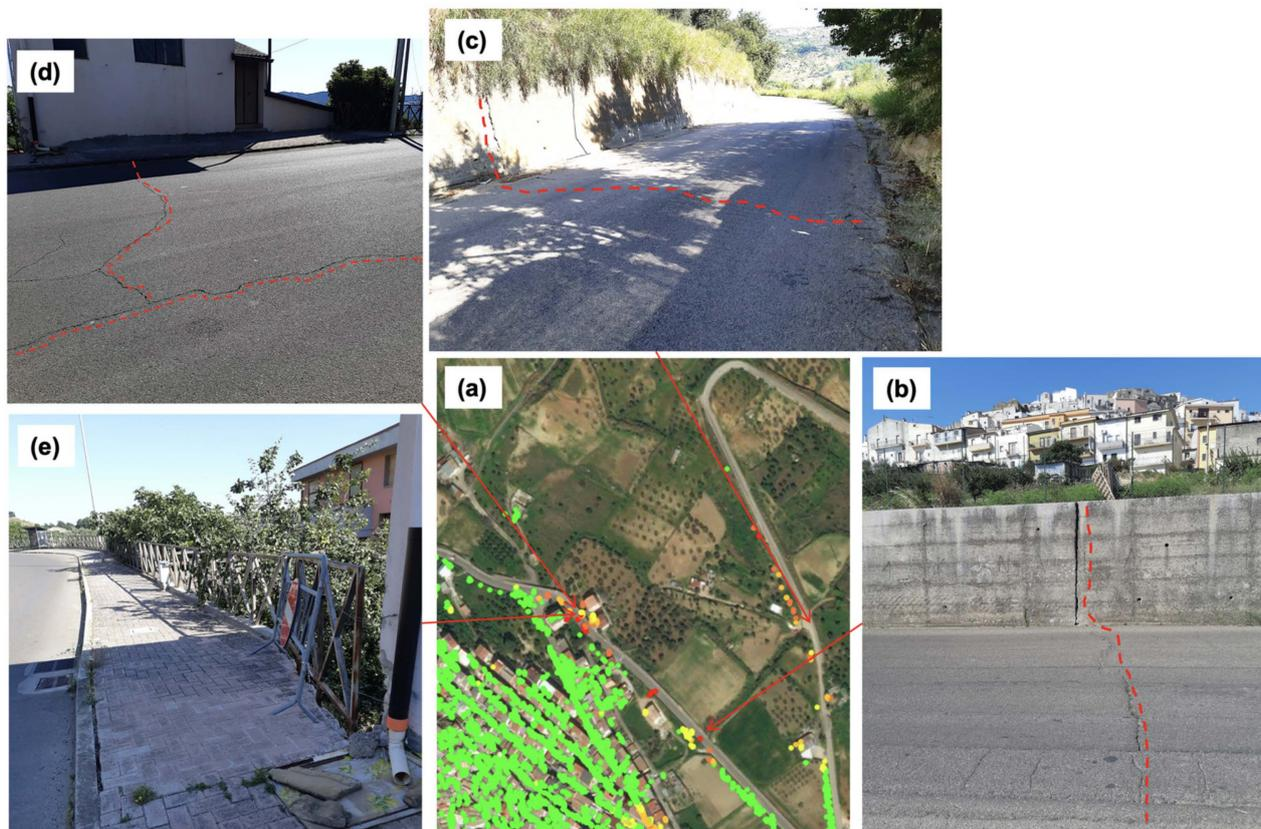
**Figure 11.** (a) Enlargement of the mean LOS S1 ascending PS displacement map of the Pomarico NE side area (same area as Figure 9a); (b–e) ground pictures of (b) cracks on the retaining wall and on the road upstream, (c) cracks on the retaining wall and on the road downstream, (d) cracks on the road, (e) damaged sidewalk.
