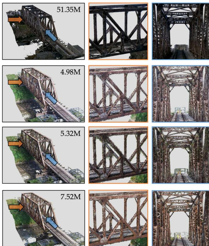
**Figure 13.** The full-bridge view (first column) with the number of points (M: Million) and the detailed views (second, third columns) of the final reconstruction of the real-world truss bridge. First row: TLS; second row: Zheng et al. [23] (Routes 1 and 3 only); third row: Zheng et al. [23]; and fourth row: Ours.
