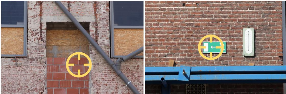
**Figure 4.** Two examples of Ground Control Points (GCPs). Because only distinctive features are selected as GCP, materialisation of the points has become obsolete.
