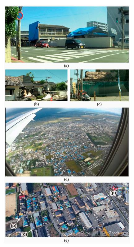
**Figure 2.** Situations of post-earthquake Kumamoto city. (a) Damaged buildings are covered with plastic sheets, whereas (b) catastrophic and (c) older buildings are neglected. (d) Roofs covered with plastic sheets are identifiable from an airplane and (e) in Google Earth 3D models. (p) Other external materials and (q) lined walls are also covered with the sheet.
