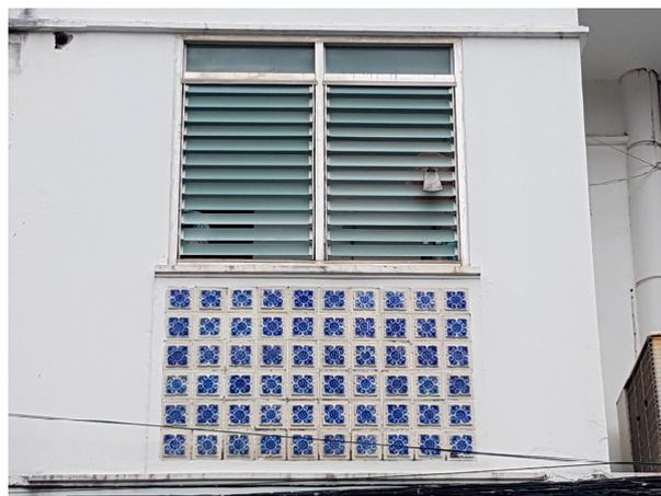
Figure 4. Typical example of louvre windows used for housing developments in urban areas of Thailand.
