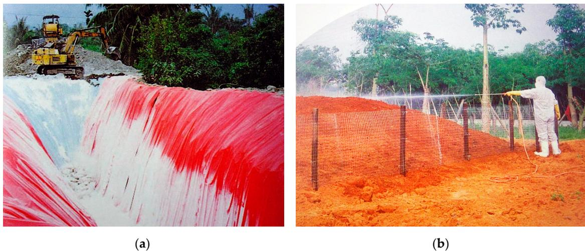
**Figure 4.** Disposal of foot and mouth disease-infected pig carcasses by landfilling with plastic liner and lime addition (a); the disposal site covered with clean soil (b).
