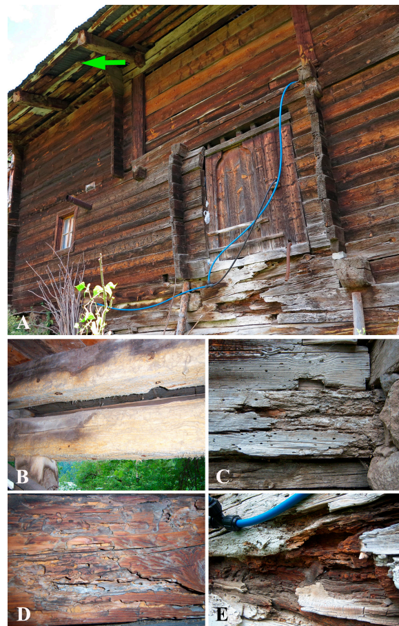
Figure 6. The wooden house damaged by old-house borer ( Hylotrupes bajulus ) and brown rot fungi. The arrow shows damaged rafter by fungi (A); Decayed wood elements in contact with water leaking (B); The wooden elements and insects in contact with the stone chimney damaged by both fungi (C); The tunnels formed by insects on the wooden wall inside the building (D); Bonding timbers near the foundation damaged by both fungi and insects (E).
