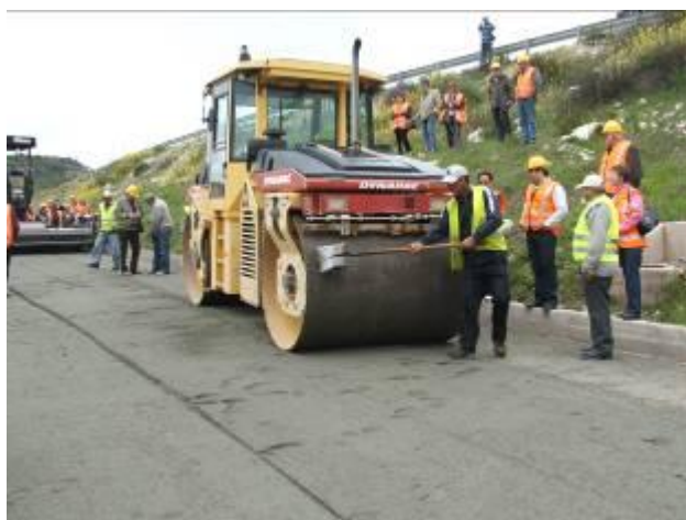
Figure 5. Roller compaction of the steel-fibre-reinforced roller-compacted concrete (SFR-RCC) layer [18].
