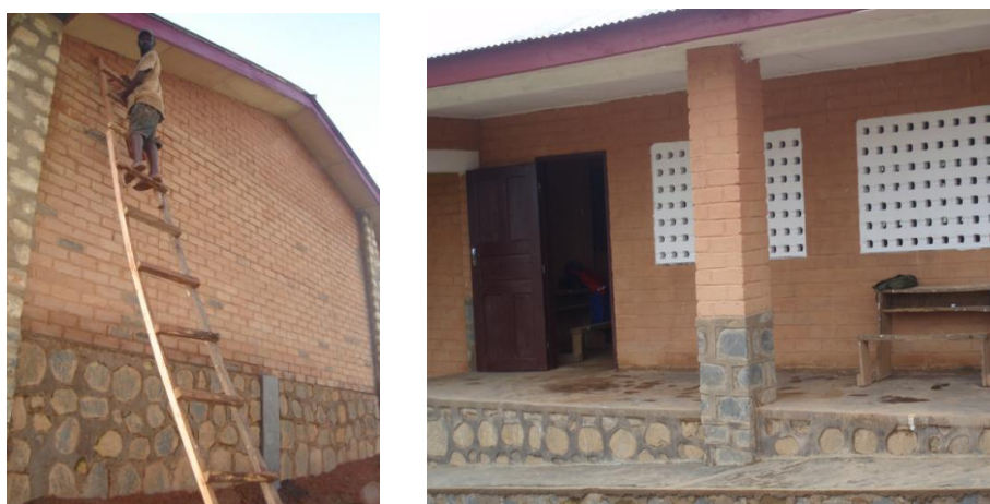
Figure 6. Two photos of classrooms with stone and Compressed Earth Blocks (CEB) with good implementation: MIPROMALO’s realization, Cameroon.
