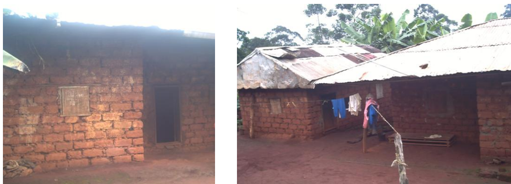
Figure 6. Two photos of classrooms with stone and Compressed Earth Blocks (CEB) with good implementation: MIPROMALO’s realization, Cameroon.
