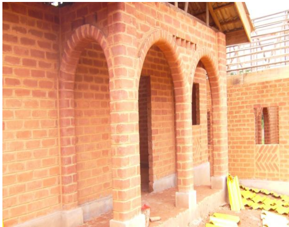
Figure 7. (a) CEB construction in Cameroon; and (b) Adobe construction in the USA.
