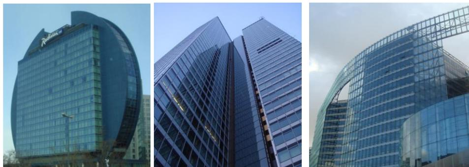
In addition, the use of these systems is very popular for renovation of non-insulated buildings. Aluminium is often used in rehabilitation works as an innovative solution that provides many advantages in restoration activities due to the exploitation of aluminium alloys' special features. Aluminium based cladding systems are durable and achieve high levels of thermal insulation and air tightness regarding external refurbishment of historical building (Figure 2).
