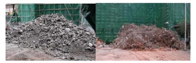
Figure 3. Sorted broken concrete and steel stockpiled separately [12].
